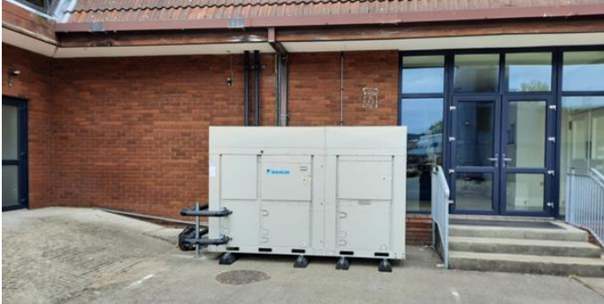
Figure 6: New Heat Pump and window replacement
